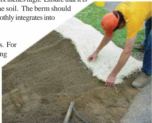
Erosion control matting made of coconut fiber is carefully placed along the berm to prevent erosion on the down hill side of the rain garden.
